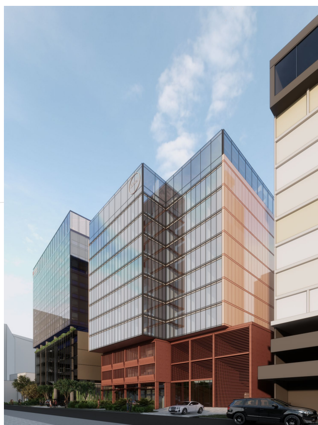
FIGURE 3 VIEW WEST ALONG BAXTER ROAD Source: Rothe Lowman 2023
