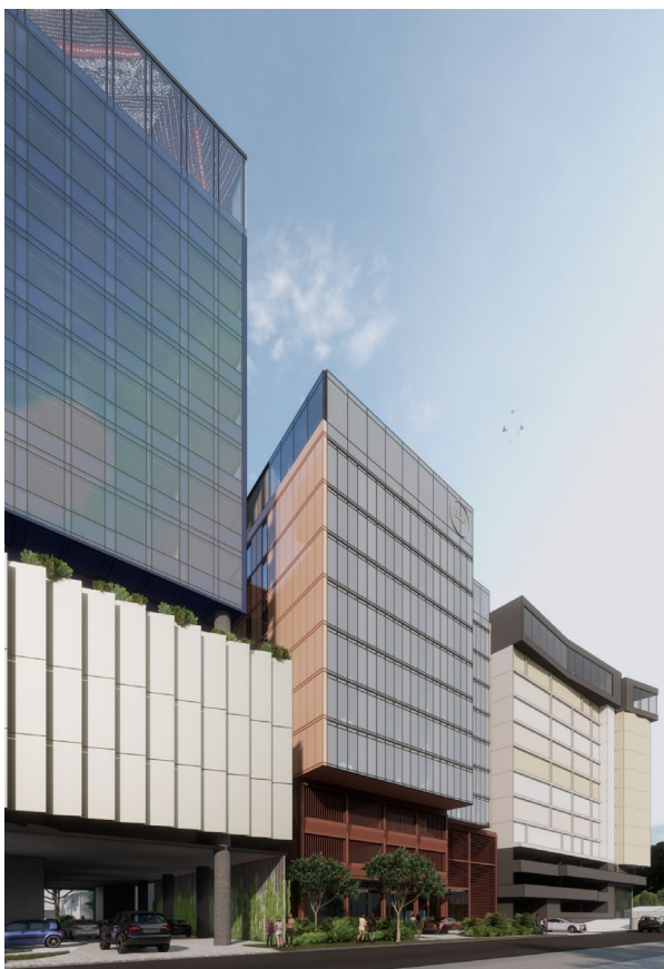
FIGURE 2 VIEW EAST ALONG BAXTER ROAD Source: Rothe Lowman 2023
